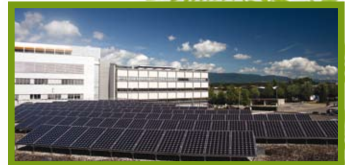
Recently installed solar panels on a roof at our Corporate Headquarters in Geneva, Switzerland.
